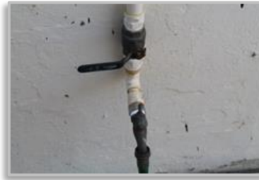
Figure 13: AV32 Spigot without Backflow Prevention Device
