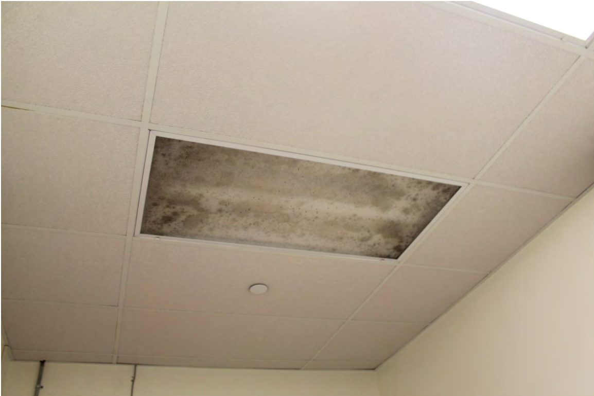
Photo 5: Visible suspect microbial growth in ceiling light cover in AV29.
