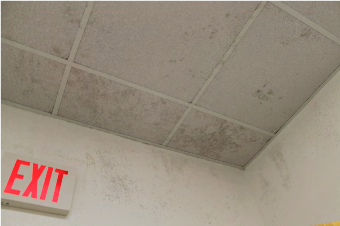
Photo 7: Visible suspect microbial growth in AV34 QRF ceiling area.
