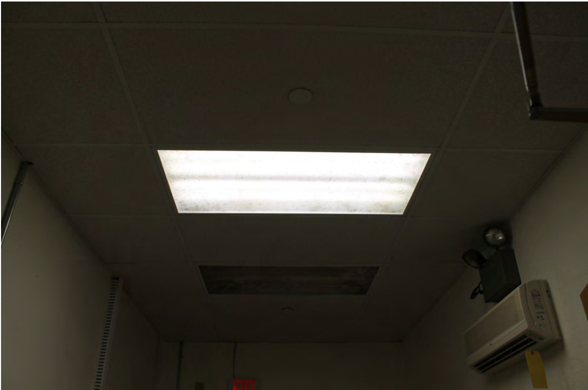
Photo 6: Condensation in ceiling light over in AV34.
