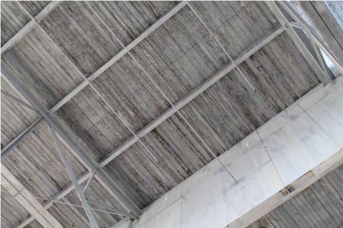
Photo 1: Scaling paint on AV32 ceiling.
