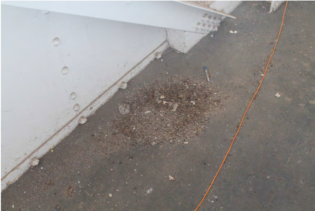
Photo 3: AV 32 mezzanine -pile of loose paint chips and other debris.
