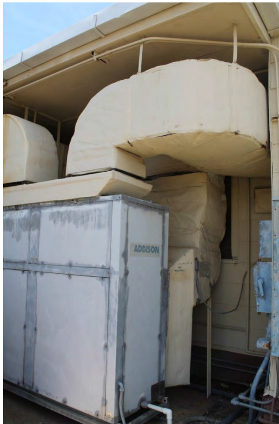
Photo 4: AV29 first floor air handling unit.
