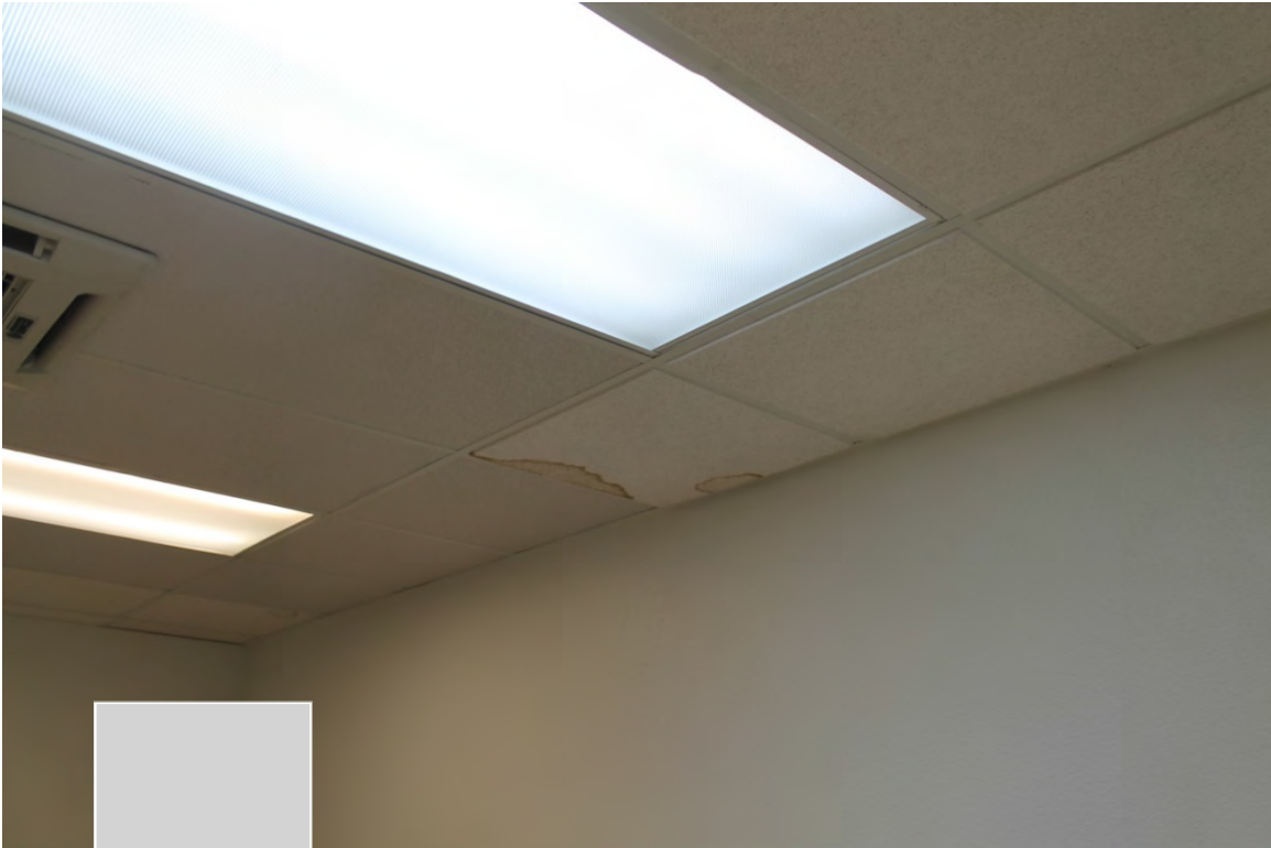
Photo 9: Stained ceiling tiles in detainee area of AV34.
