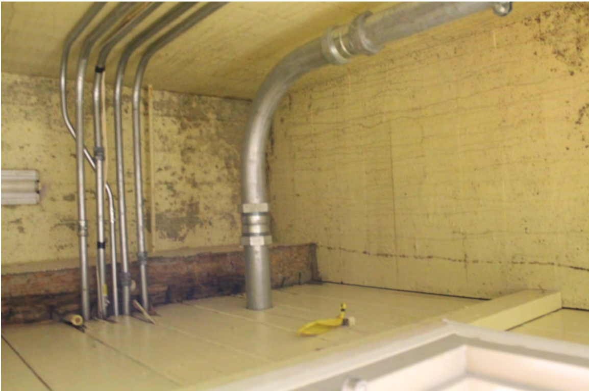
Photo 8: Visible suspect microbial growth in AV29 closet
