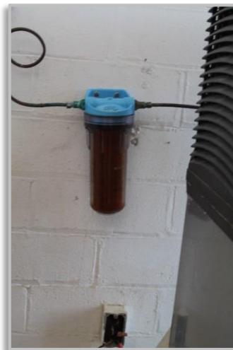
Figure 15: AV32 Bulk Ice Machine Water Filter
