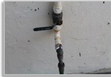
Figure 13: AV32 Spigot without Backflow Prevention Device
