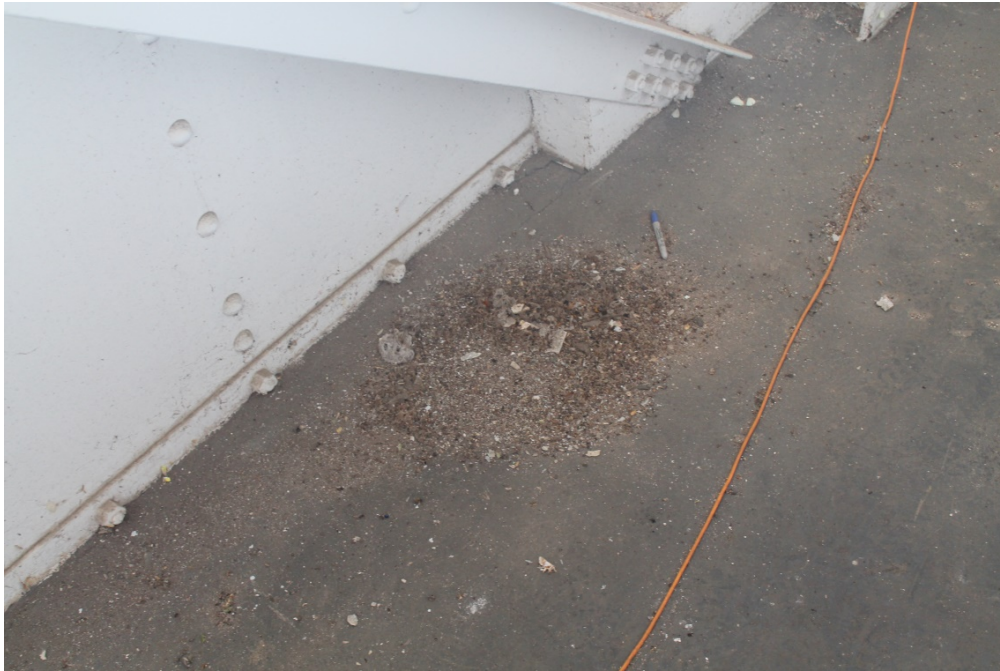
Photograph 3: AV32 mezzanine-pile of loose paint chips and other debris.
