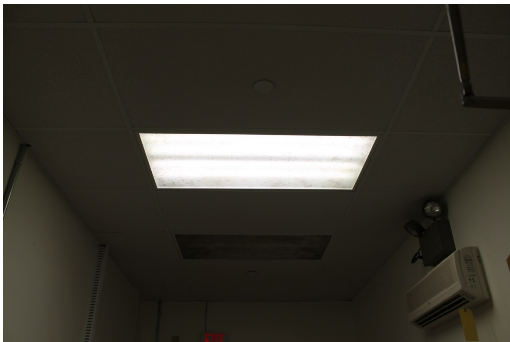
Photograph 6: Condensation in ceiling light cover in AV34.
