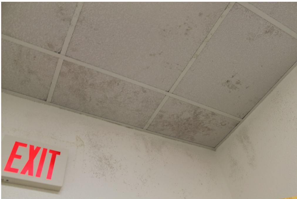
Photograph 7: Visible suspect microbial growth in AV34 ceiling area.
