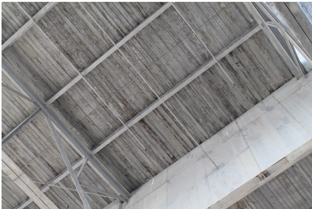
Photograph 1: Scaling paint on AV32 ceiling.
