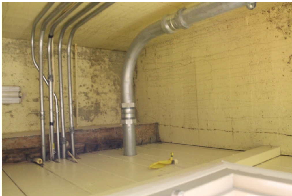
Photograph 8: Visible suspect microbial growth in AV29 closet
