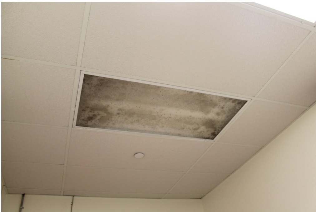
Photograph 5: Visible suspect microbial growth in ceiling light cover in AV29.
