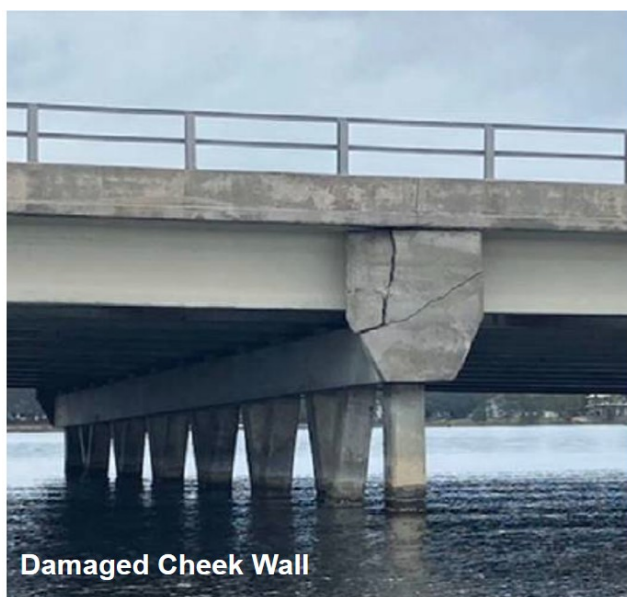
Figure 4-1. Damaged Cheek Wall on the Main Gate Bridge
