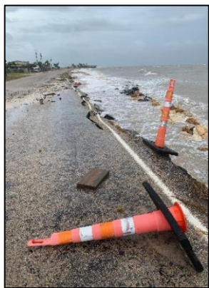
Highway 316 in Indianola, TX. Image – TX DOT
