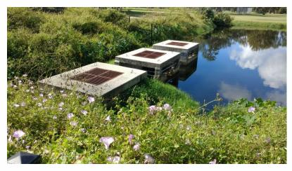
A **STORM** sewer system in which the flow receives little to no treatment prior to flowing into the river. Storm sewer lines are typically comprised of metal or concrete culverts and pipes, concrete or grass lined ditches, and catch basins (inlets).
