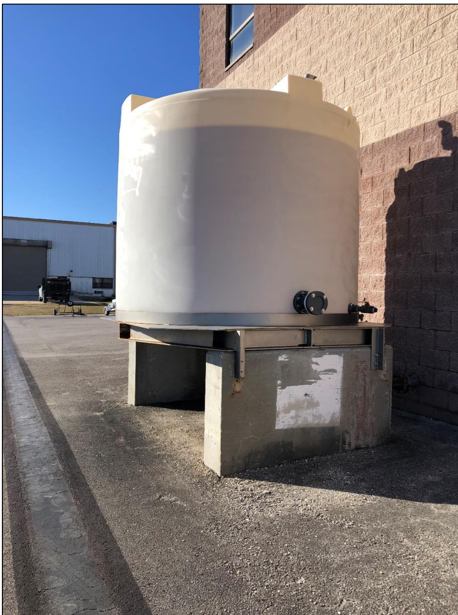
Unlabeled fire suppression AST (single-walled).
