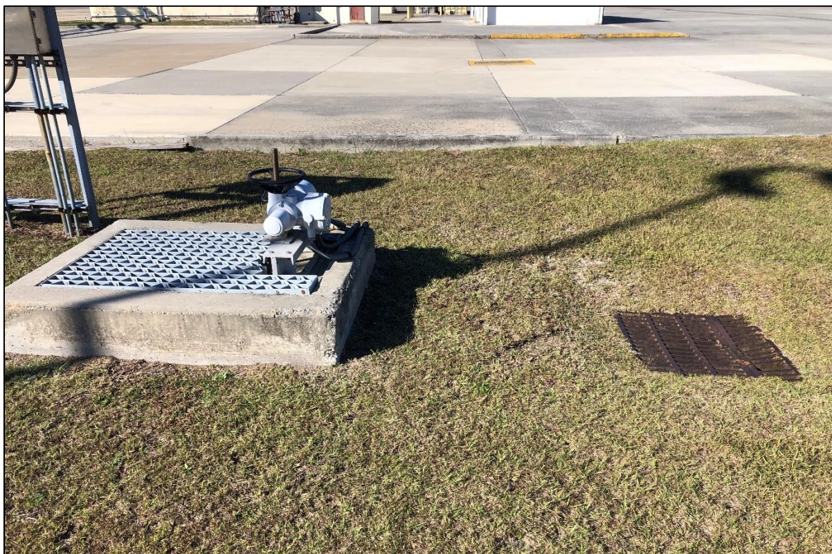
Aircraft wash rack diversion valve system was inoperable (all flows diverted to sanitary sewer).
