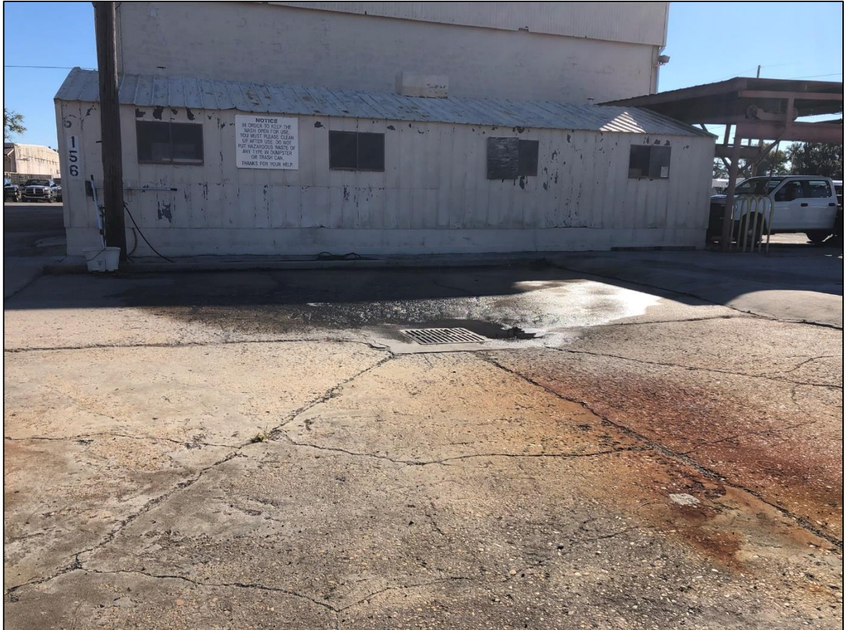
Cracks in vehicle wash rack concrete pad.
