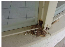
Drywood termite damage
