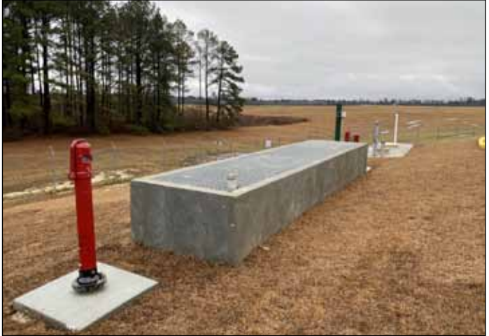
Submitted photo The new oil water separator will increase the operational capacity of the fuel facility onboard NAS Meridian.
