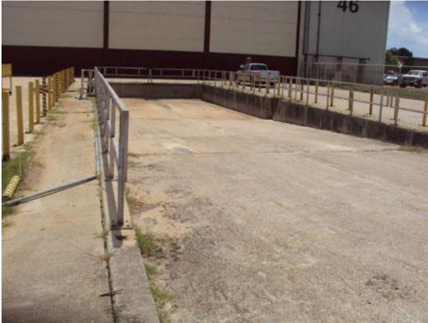
(1) Loading dock at hangar 46.
