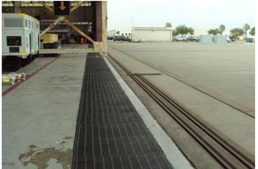
(2) Hangar door with internal drain
