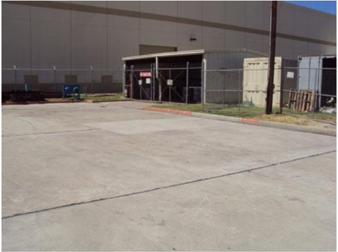
Wash rack and hazardous waste area associated with Hangar 56.
