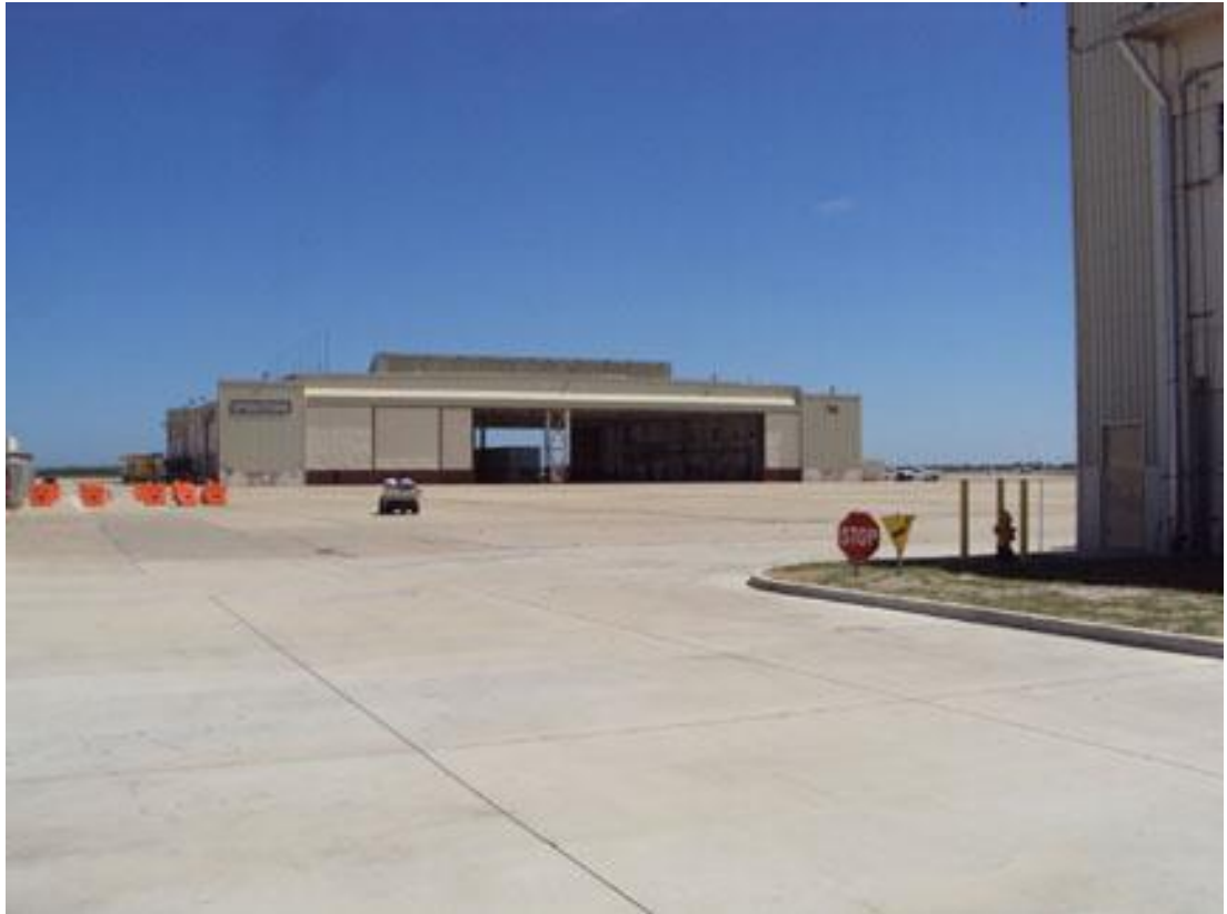
Hangar 58 empty. Construction finished.
