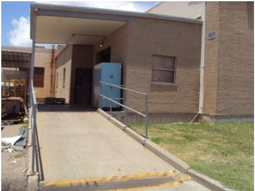
(1) Covered loading dock
