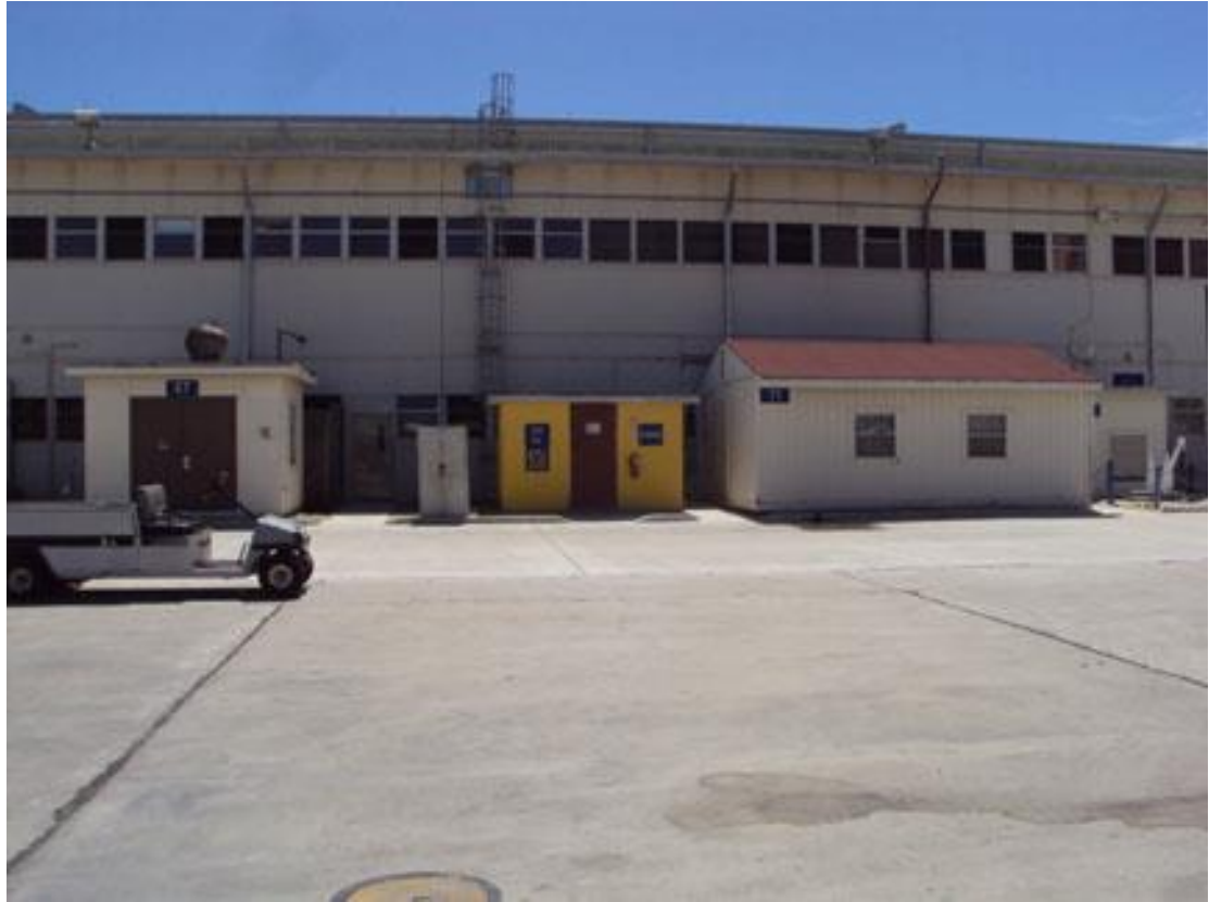
Flammables locker associated with Hangar 57.
